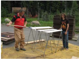
Niel Barrett & Branden Marlow painting siding.
