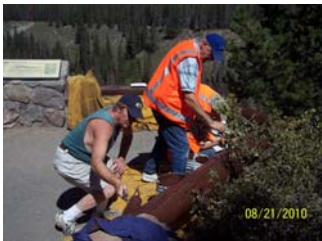
Rick Foster, Robert Marlow painting log railing at Pinnacles.
