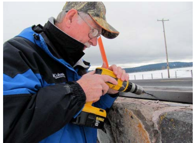
Dave Panebaker drilling.
